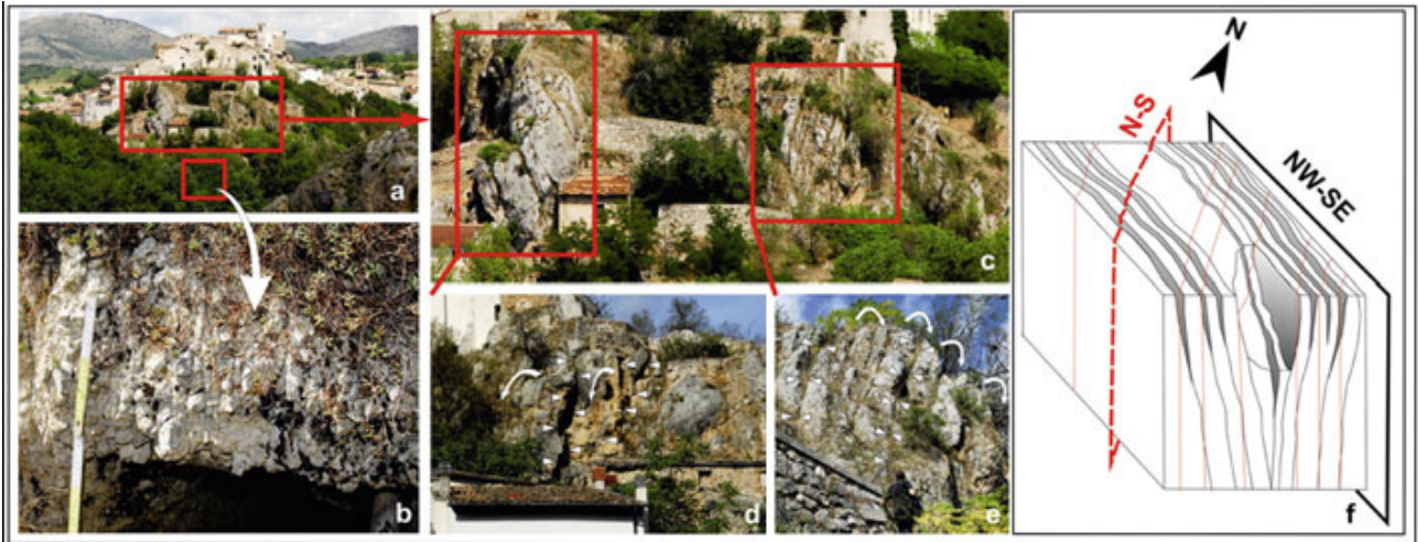
Figure 3. a Panoramic view of the southern termination of the Castelvechio Subequo ridge; b close-up photograph showing narrowly spaced shear planes and closed fractures affecting the limestone bedrock at the lowermost portion of the ridge; c close-up image of the uppermost portion of the ridge, where opening mode discontinuities affect the carbonate bedrock; details of the open fractures (indicated by white triangles ) detected along the western d and eastern e flanks of the ridge; white arrows indicate the direction of toppling of the bedrock slabs; f block diagram showing the main sets of fractures affecting the Castelvechio Subequo ridge (from Marzorati et al., 2011).
