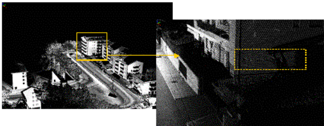
Figure 9. A damaged edifice and a detail of the cracks.
