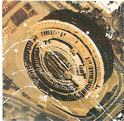
Fig. 3. An aerial view of the Colosseum showing the perfect coincidence between the trend of the Fosso Labicano Valley and the southern portion of the monument, where nearly all the damage is concentrated. Dashed lines indicate the limits of alluvial deposits. Dots indicate the location of drillings that provided data for the investigation of the local stratigraphy. A-A': location of the restored portion of the inner ring.
