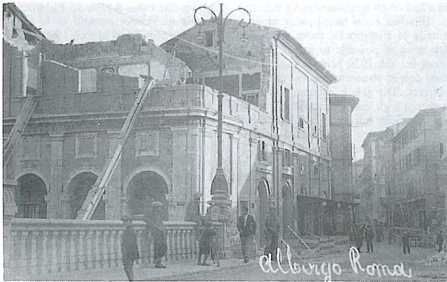
Fig. 4. The «Albergo Roma» after the 1930 quake. Located along the Misa river, it had its second floor completely destroyed.
