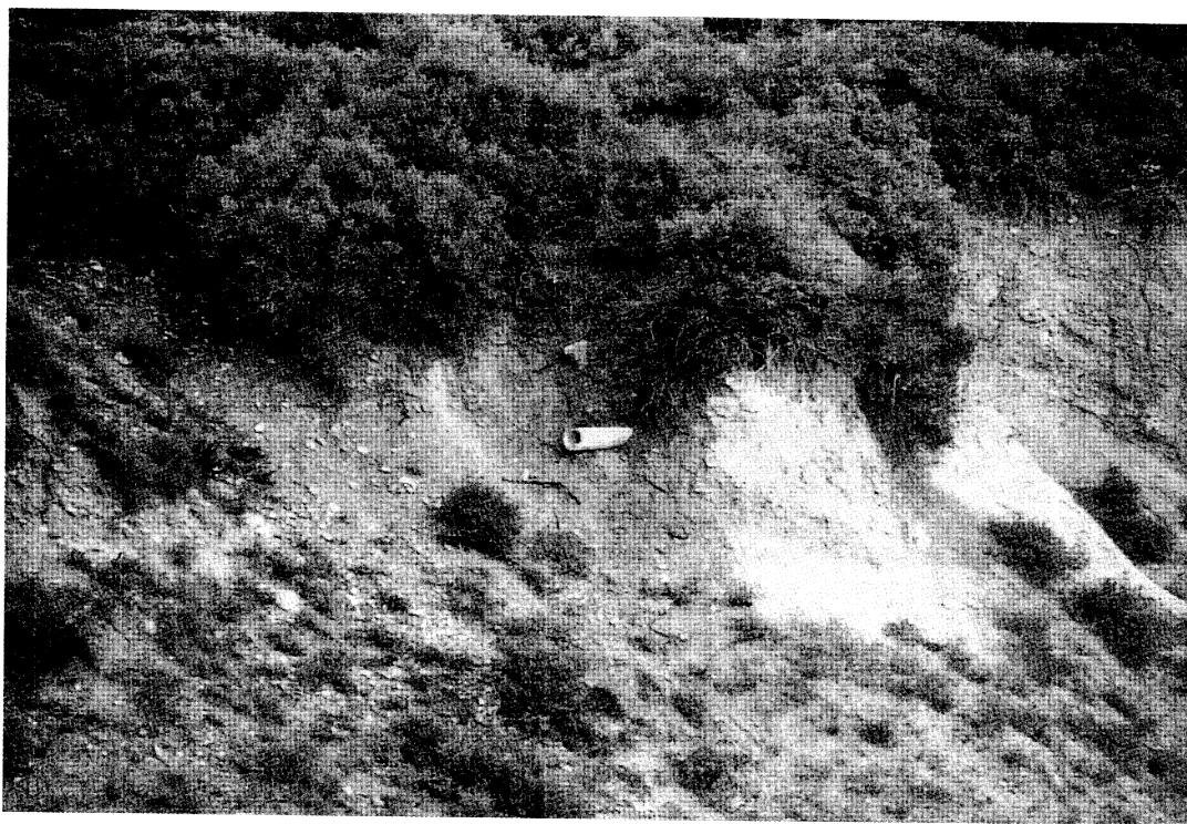
Fig. 5. The palaeochristian aqueduct buried 1 m deep, which crops out along the eastern flank of a N-S trending stream entrenching the foot-wall block of the NAFS (site b in fig. 2). A similar setting has been observed on the other side of the valley.
