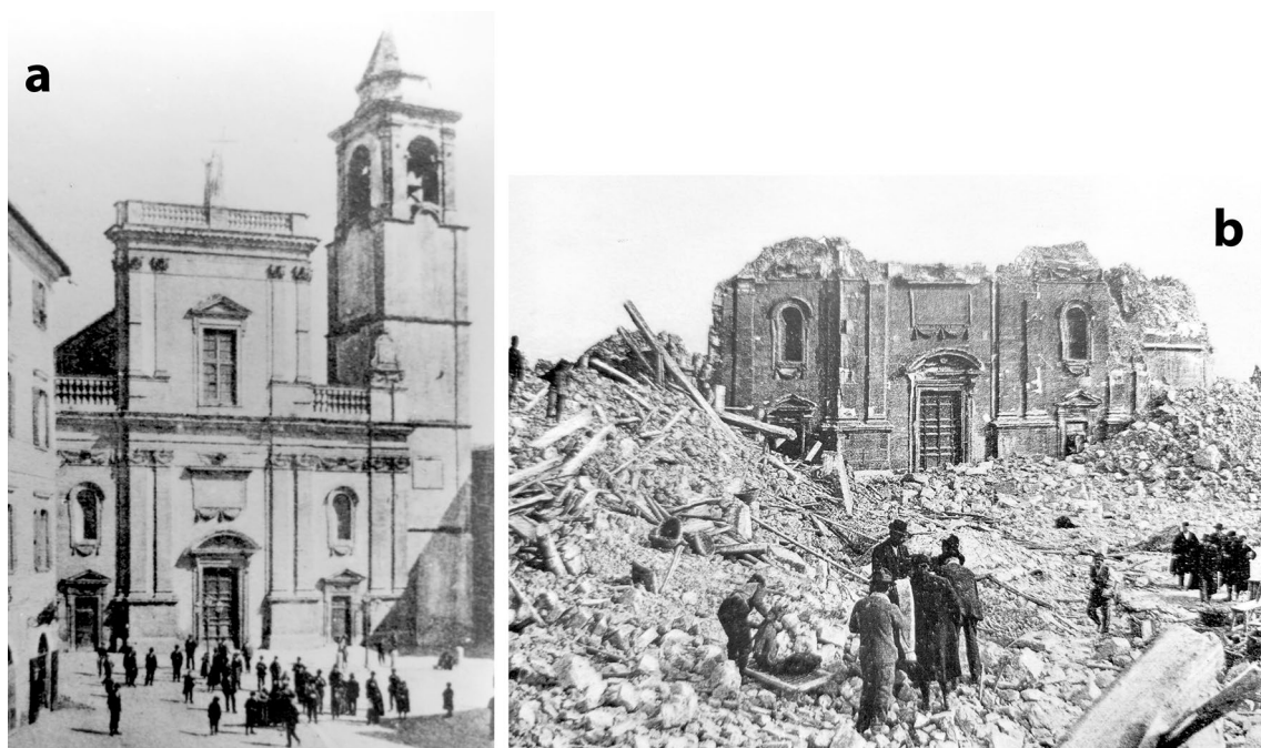
Fig. 11 Avezzano, church of San Bartolomeo (16th–17th century) before (a) and after (b) the 1915 earthquake (historical photos from personal archive of F. Galadini)
