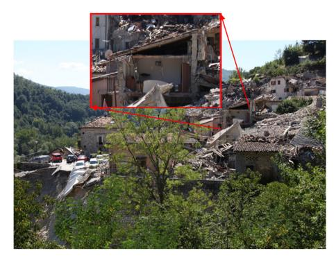
**Figure 3.** Exploration of a snapshot by AR. The augmented information highlights in red the state of the damage within the buildings at Pescara del Tronto after the earthquakes in central Italy in August 2016 (photo credits: Raffaele Azzaro).
