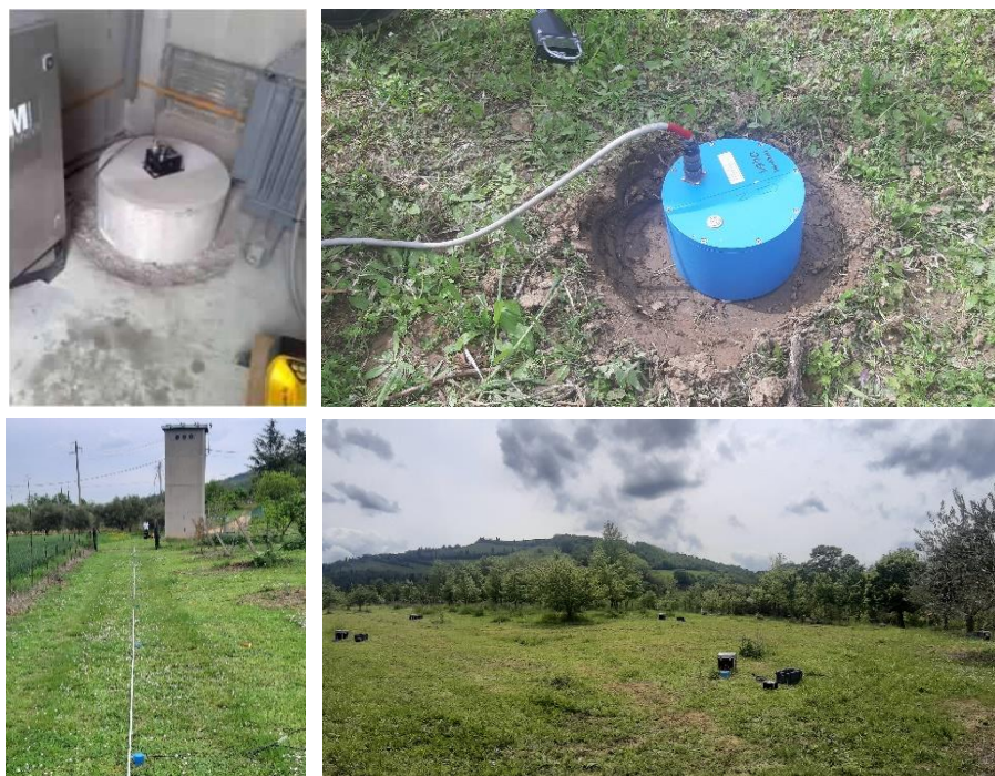
Figure 7: Upper left: accelerometric station IT.BRH installed in Brisighella (RA). Bottom left: ENEL transformer cabin where the station IT.BRH is installed and MASW acquisition line. Upper right: single station ambient noise measurement. Bottom right: 2D passive ambient noise array installed close to the IT.BRH station.
