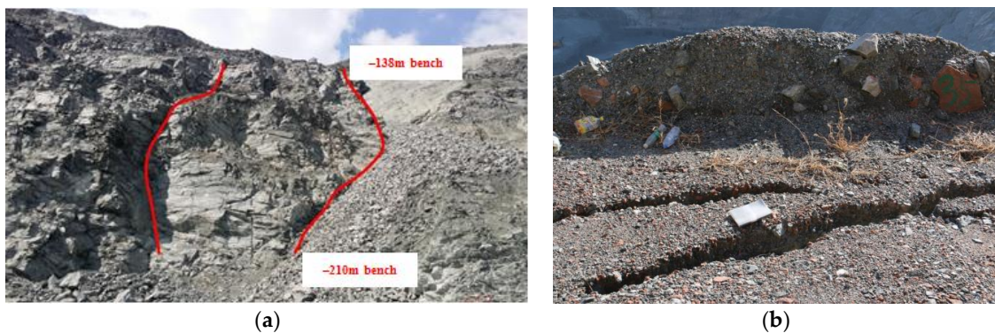
Figure 4. Photograph of the landslide on 27 May 2018: (a) left and right borders; (b) crack on the top border at -138 m bench.
