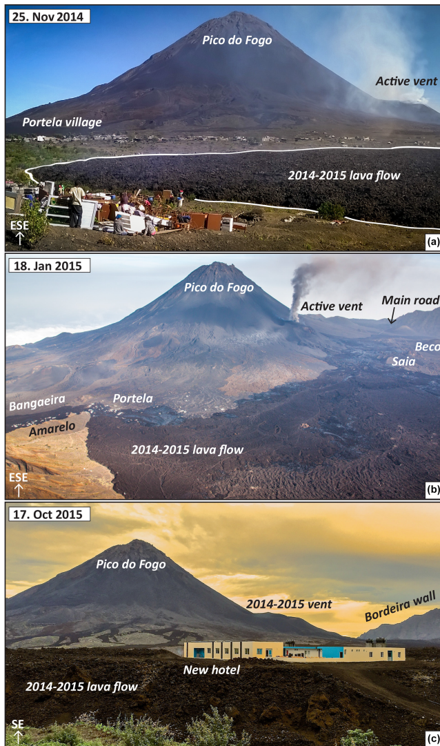
Figure 2. Photographs taken during (a and b) and after (c) the 2014–2015 Fogo eruption. On 25 November 2014, the village of Portela was not yet engulfed by lava flows, but private belongings were brought to higher ground (a), while on 18 January 2015 lava flows were covering the villages of Portela and Bangaieira (b). In early October 2015, a new hotel opened which is built on the 2014–2015 lava flow (©Mustafa Kerim Eren) (c).
