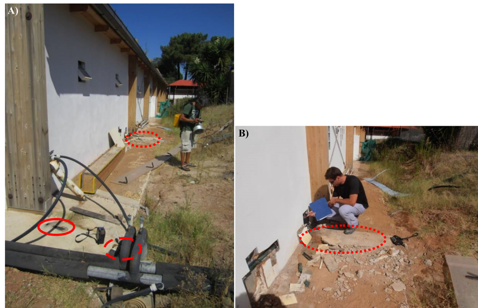
Figure 6. (a) SE corner and (b) eastern wall of the building hosting the service rooms of the Lavinio Country Club pool. Solid, hatched, and dotted red circles indicate the sites where outdoor gas air concentration was measured (results in Table 2).
