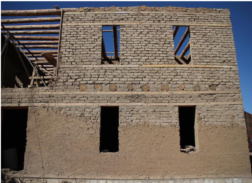
Figure 3 - Adobe house with anti-seismic presides
