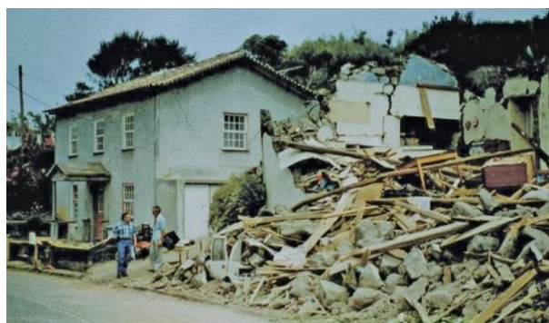
Figure 9. Difference of seismic performance between adjacent constructions
