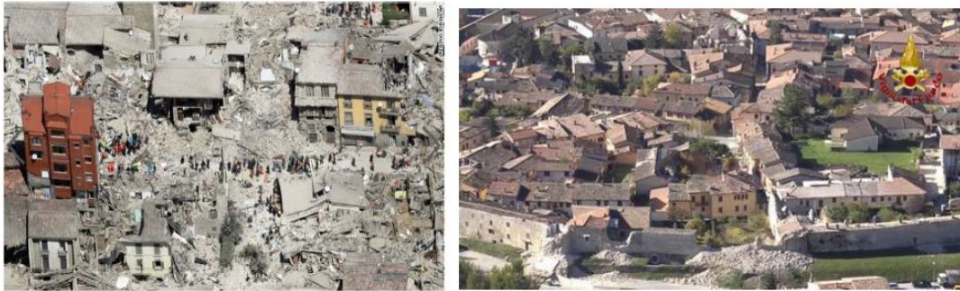
Figure 3. Left) Amatrice after the August 24 th earthquake. Right) Norcia after the October 30 th 2016 earthquake
