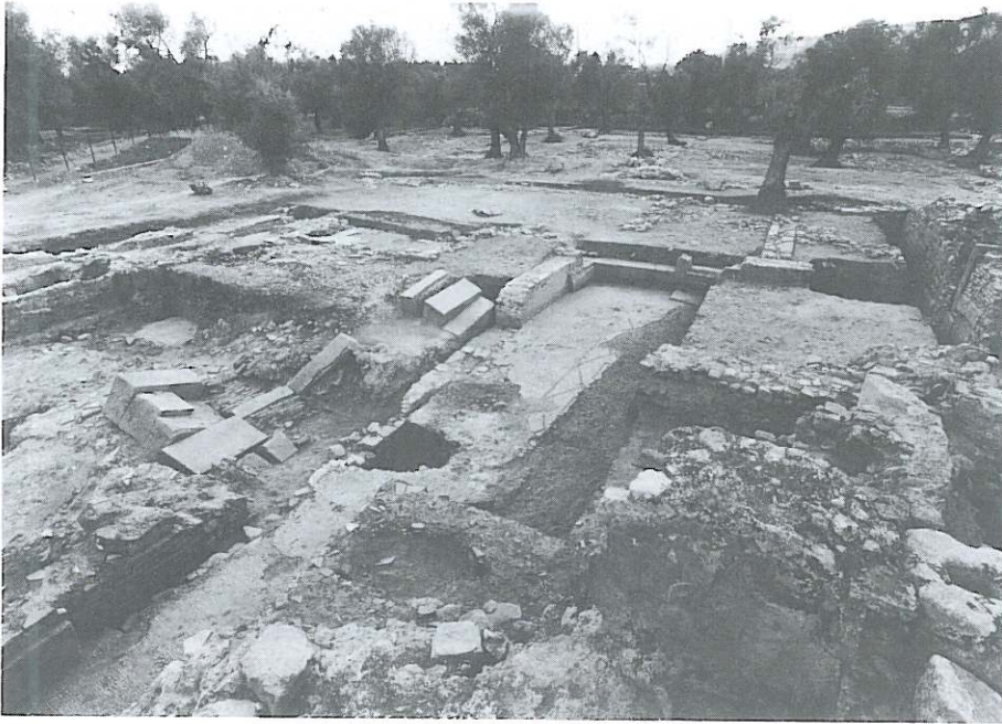
Fig. 5. Gortyn (Crete) Praetorium , rooms 45 and 47, the southward collapse of the US 406 wall because of the earthquake of 365 A.D. (excavations of Italian School of Archaeology in Athens, 1989-91).
