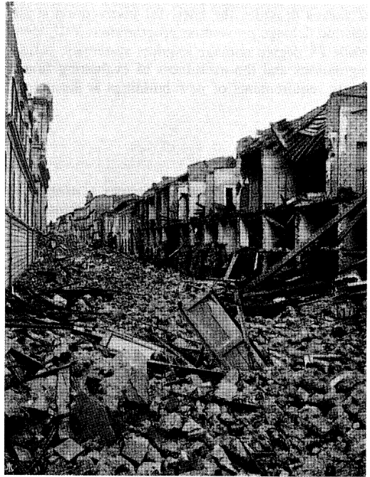
Fig. 1. The overturning of façades along a street of Messina after the earthquake (December 28th, 1908).
