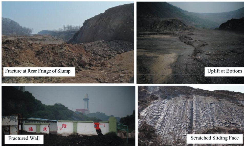
Figure 2. Landslide-induced surface phenomena.
