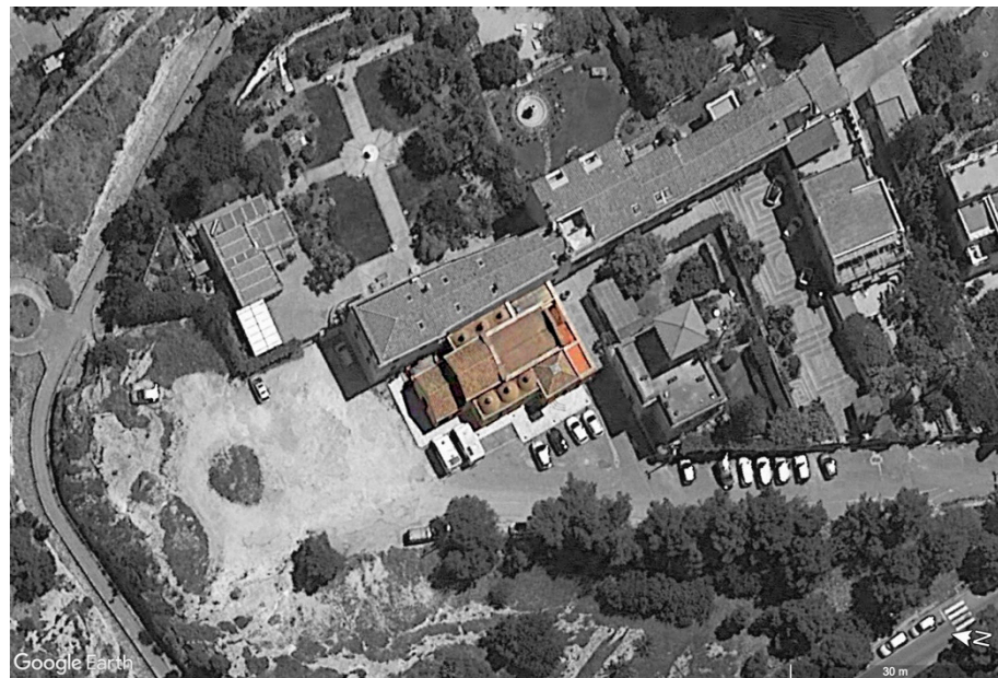
Figure 1. Aerial view of the ancient Romanesque church of Saints Lorenzo and Pancrazio, which dates from the second half of the 13th century and is located in the historical town of Cagliari (Italy) (elaborated from Google Earth).
