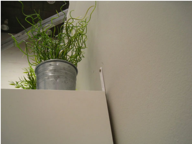
Fig. 23.8 Top-heavy furniture should be secured to a wall
