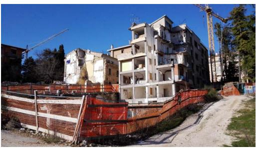
Fig. 64 - Example of RC building collapsed in Via Campo di Fossa during the April 6, 2009 main shock.
