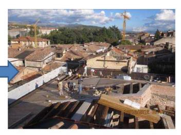
Fig. 77 - Reconstruction of the wooden roofs conserving the original configuration.
