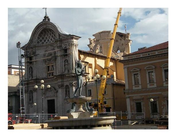
by the earthquake. church was severely damaged by the 2009 earthquake, in particular the superb dome (attributed to G. Valadier), the lantern and the spires collapsed. The transept and roofing were in danger of collapse.
