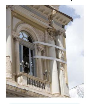
Fig. 71 - Particular of the Biblioteca Tommasi. The building was very severely damaged: the main facade was in danger of collapsing.
