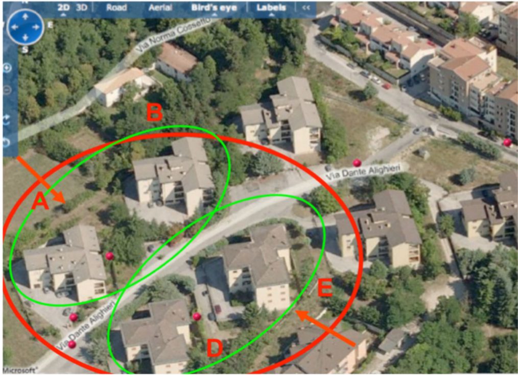
Figure 2: Aerial view of the area with the investigated buildings. Red arrows point to buildings collapsed (A and E) due to soft storey mechanism.
