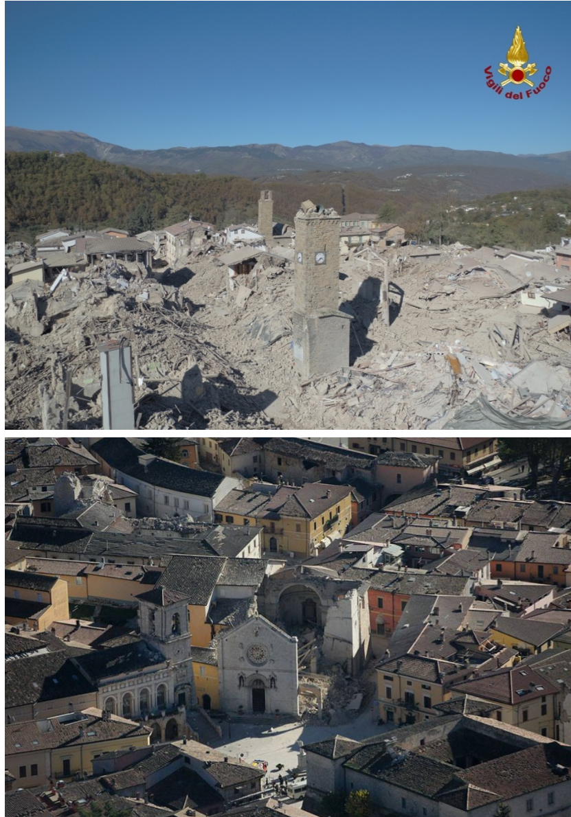
Figure 2 – Aerial views of Amatrice and Norcia taken at the beginning of November 2016. In Amatrice (above) very few buildings were left standing by the combined effect of the 24 August and 30 October shocks. In Norcia, (below) the 30 October shock wrecked most of the St. Benedict church (its façade is still visible in the middle of the picture), but the rest of the town appears largely unscathed, including the Palazzo Comunale (Town Hall), located to the left of the church, along with its superb clock tower.
